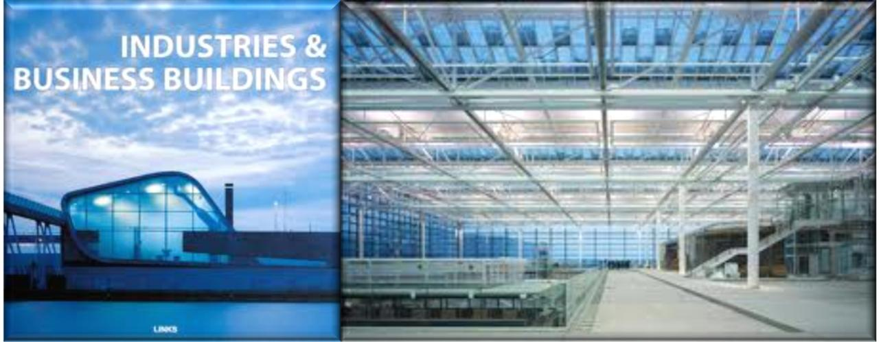
The use of steel structures in industrial constructions meets the architectural needs most appropriately. Large apertures, local-variable definitions and variable load sizes are some of the main reasons why steel is preferred as the main structure of industrial constructions.
